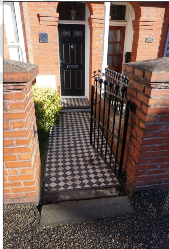
Fig. 15: Geometric tiled path leading to panelled door with decorative glass feature and fan light window.
