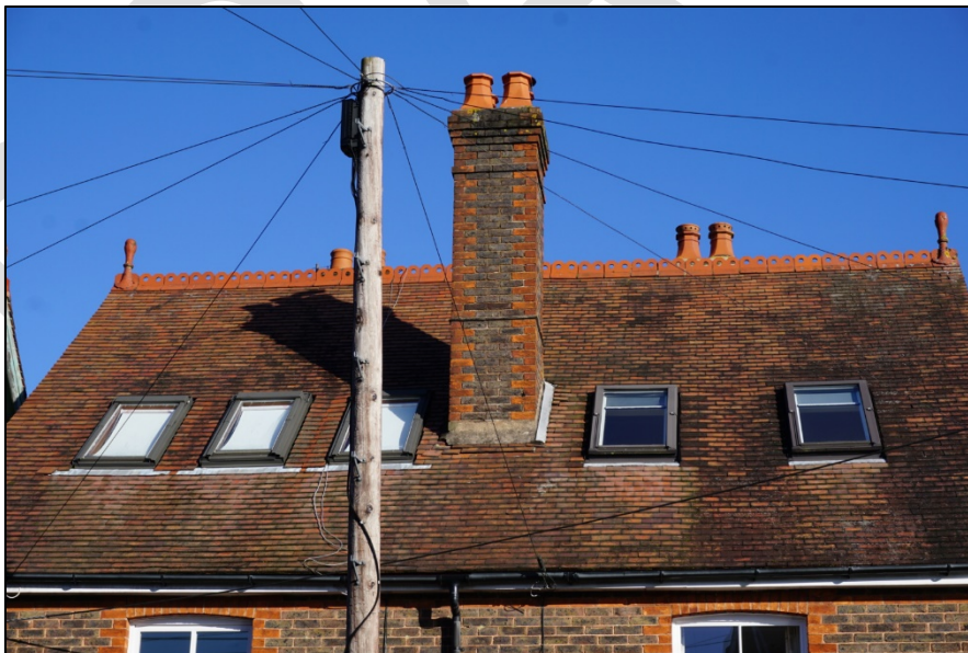
Fig. 10: Two hole hexagonal crest ridge tiling with finials and red brick chimney stack quoin, Hazelwick Road.
