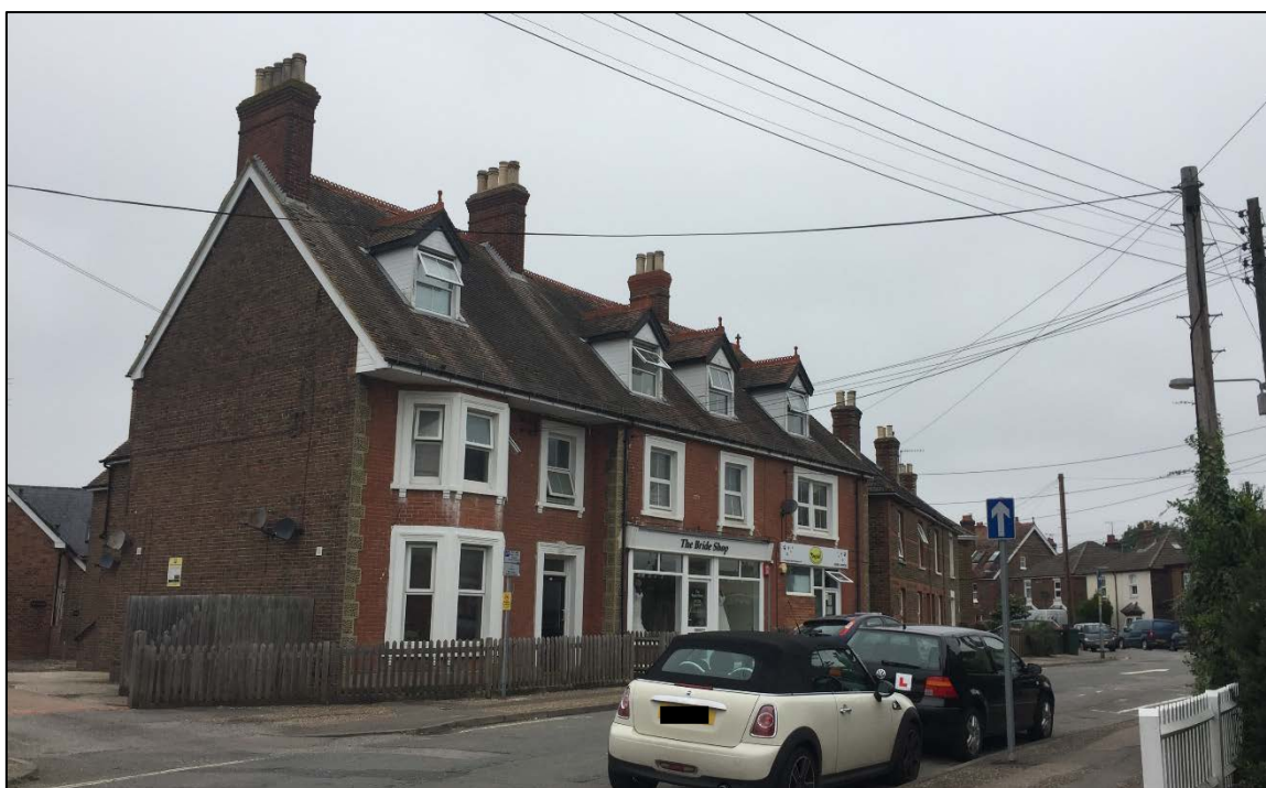
Fig. 24: The terraced building at 52-54 Hazelwick Road makes for a prominent presence at the conservation area midpoint.
