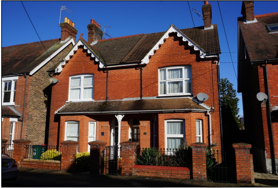
Fig. 14: Projecting porch with slate tiled roof and period detailing. Note also the low level boundary brick wall with capped piers and railings.
